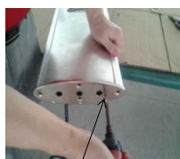
24 Nineteenth step: install the under damper.
