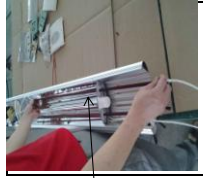
2 install heating element 2.
