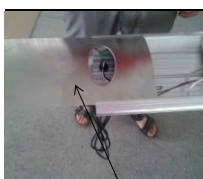
21 Sixteenth step: install PCB box protection board.
