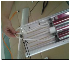
12 Twelfth step:pull the wire's terminal out.
